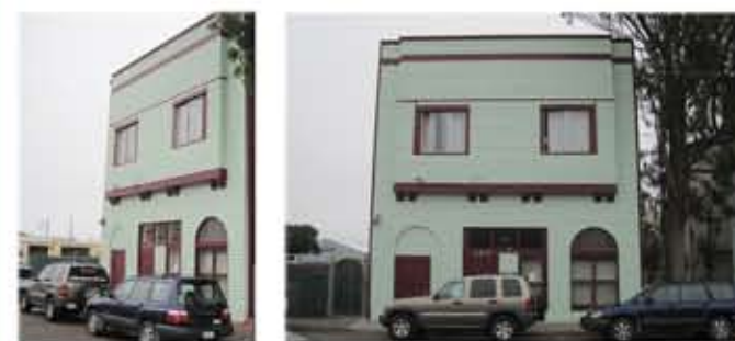
Fresh paint at the Women & Children's Shelter
